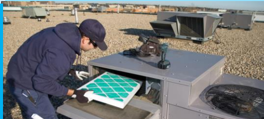
Ventilation System Maintenance
